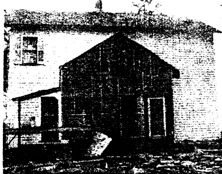
Silhouette of demolished building
